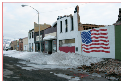
San Marin Hotel following the 2008 M 6.0 Wells, Nevada earthquake
