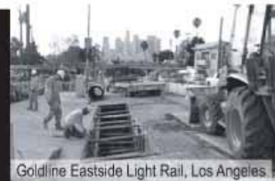
Goldline Eastside Light Rail, Los Angeles
