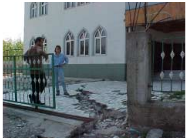
Figure 12 Fault traversing beneath the corner of the Koran School, yet the school underwent only minimal damage (Photo by E. Rathje).
