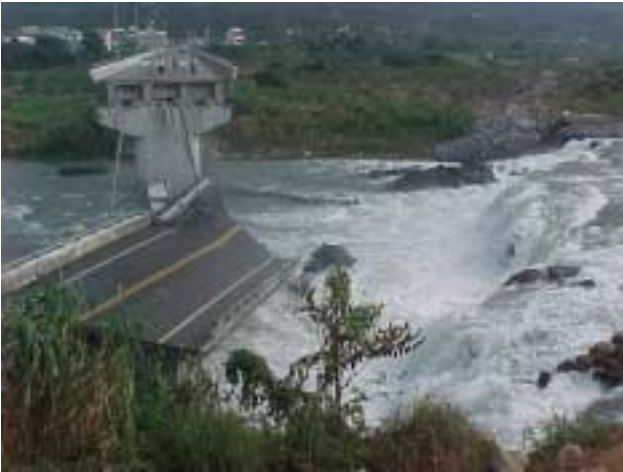
Figure 16 Collapse of Highway 13 bridge north of Fengyuan due to 6 m fault movement (Photo by J.D. Bray).
